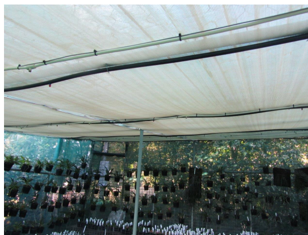
Misting and sprinkler piping beneath stone shade cloth.
