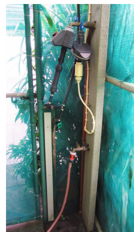
Misting and sprinkler controls on post inside shade-house door.
