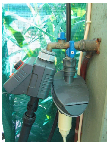
Misting timer on the right, sprinkler timer on the left.
